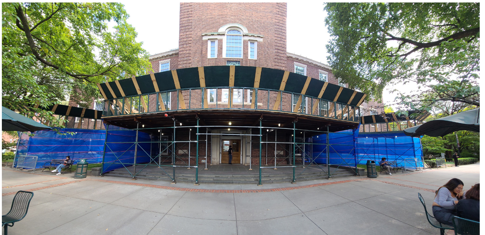
Scaffolding outside of the library./Daniel Afanasyev
